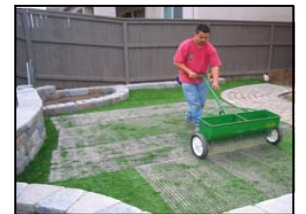
Infill Applied to Surfaces
